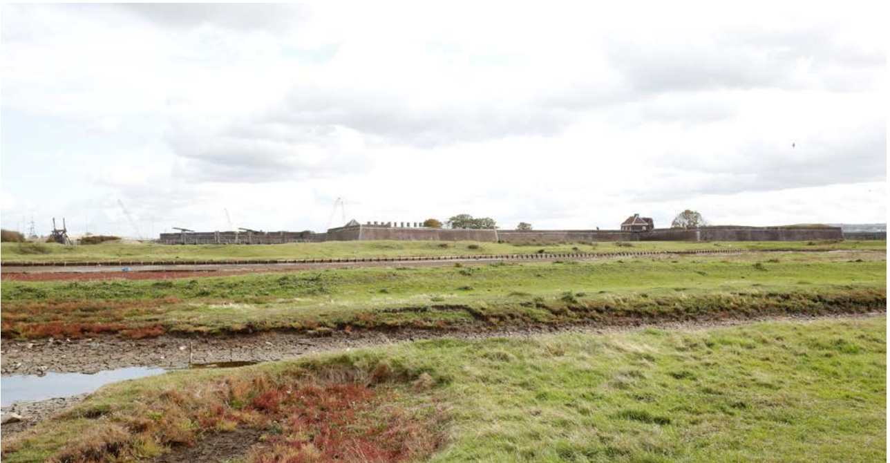
Plate TF7: View of Tilbury Fort from the north-west
