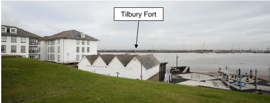
Plate NTF8: View from 6-inch gun emplacement on the angled battery looking towards Tilbury Fort
