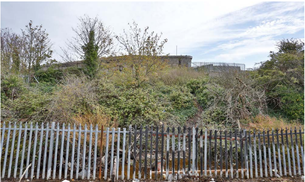
Plate CLF3: The fort obscured behind security fencing and vegetation
