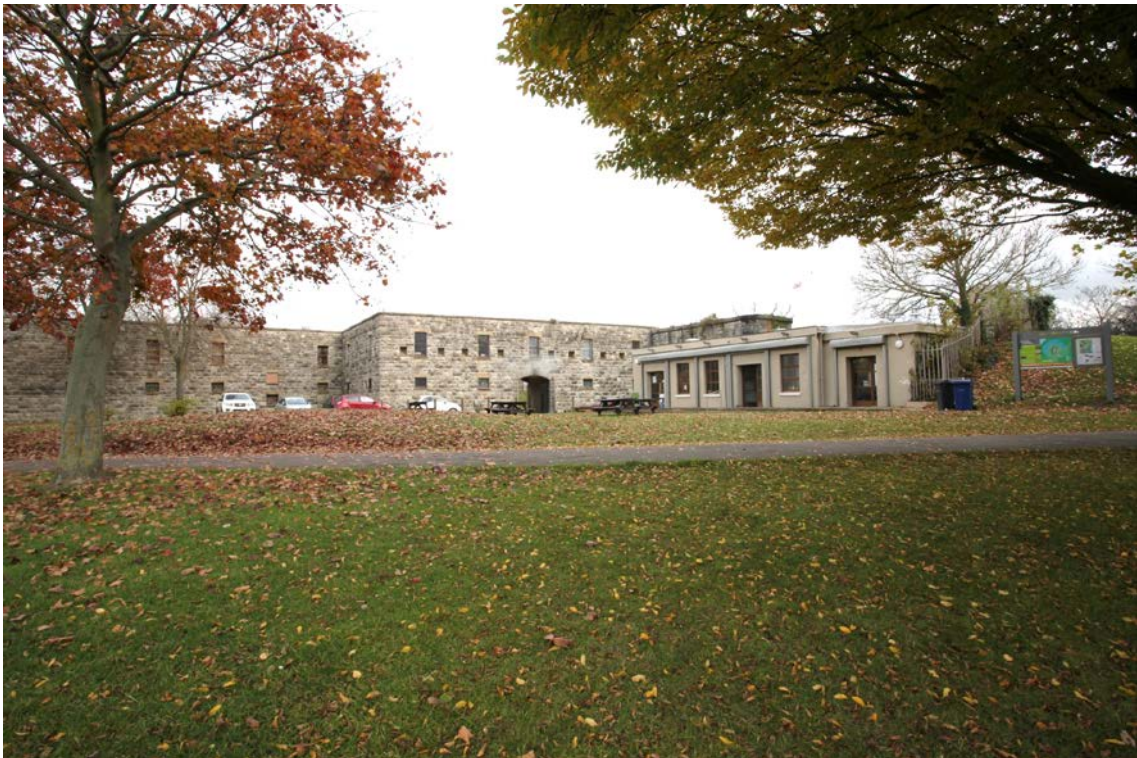
Plate CHF1: Coalhouse Fort exterior including the Generator House
