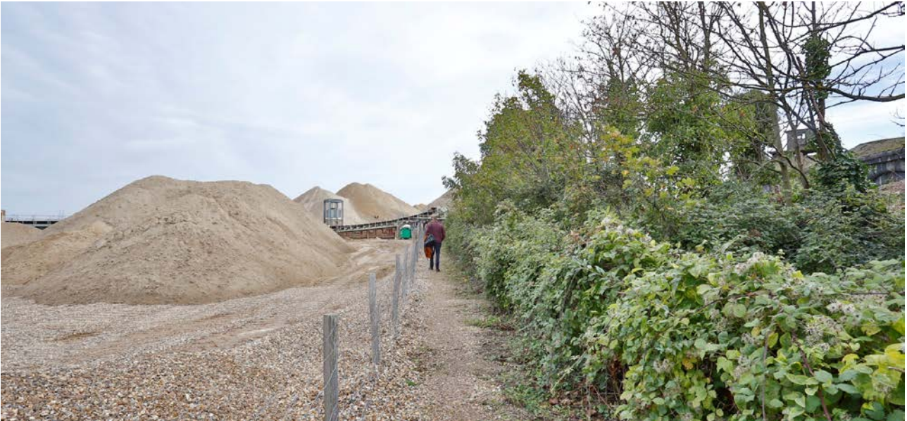
Plate CLF4: Access around the north side of the fort. The fort is partially visible on the right.
