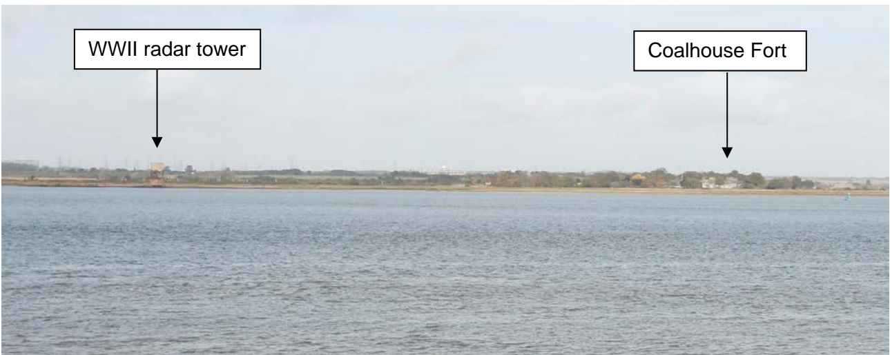
Plate CHF6: View of the Coalhouse Fort Scheduled Monument from the south side of the Thames at a point between Shornemead and Cliffe Forts
