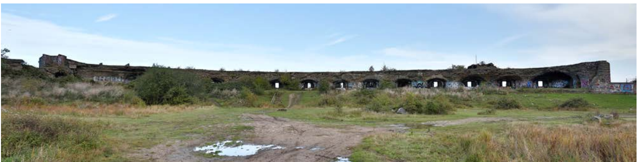
Plate SF2: Interior of the fort showing the rear of the casemate
