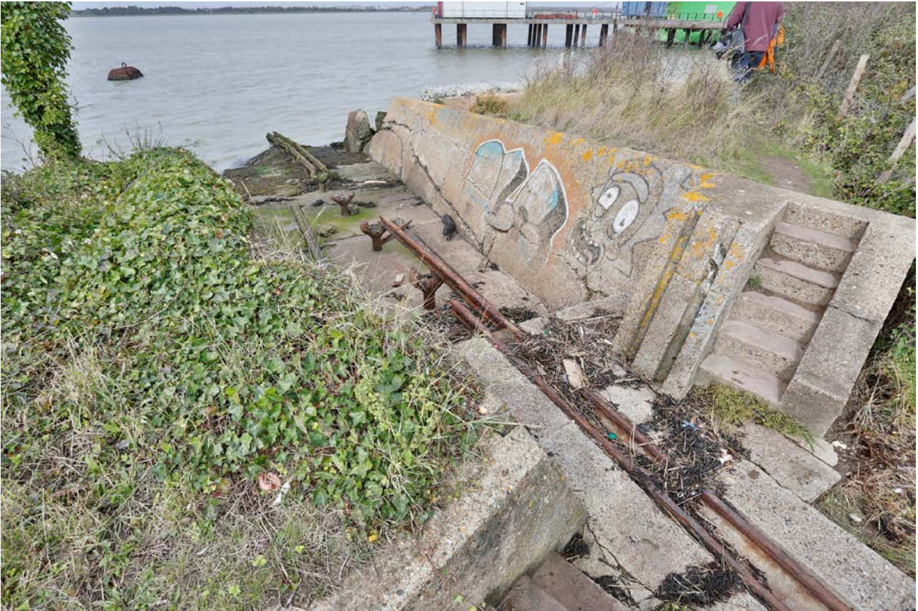
Plate CLF6: The Brennan Torpedo slipway
