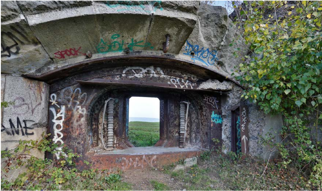
Plate SF5: Detail view of a gun emplacement showing the survival of metalwork
